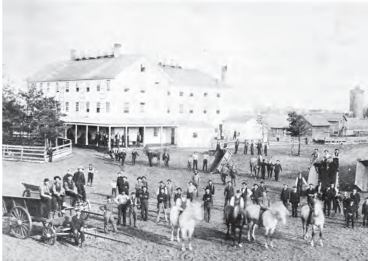
Historic Boarding House Image Source: Ford River Township
